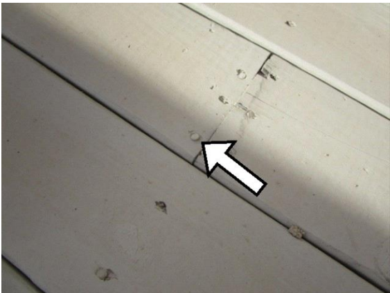
Decks / Balcony: Protruding Nails
